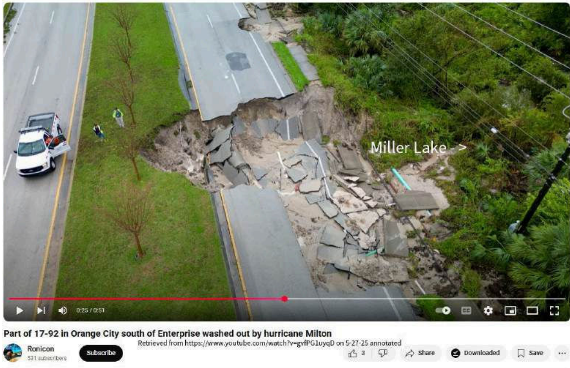
Figure 2 Water from Shadow Stormwater Destroying South Volusia Ave.
